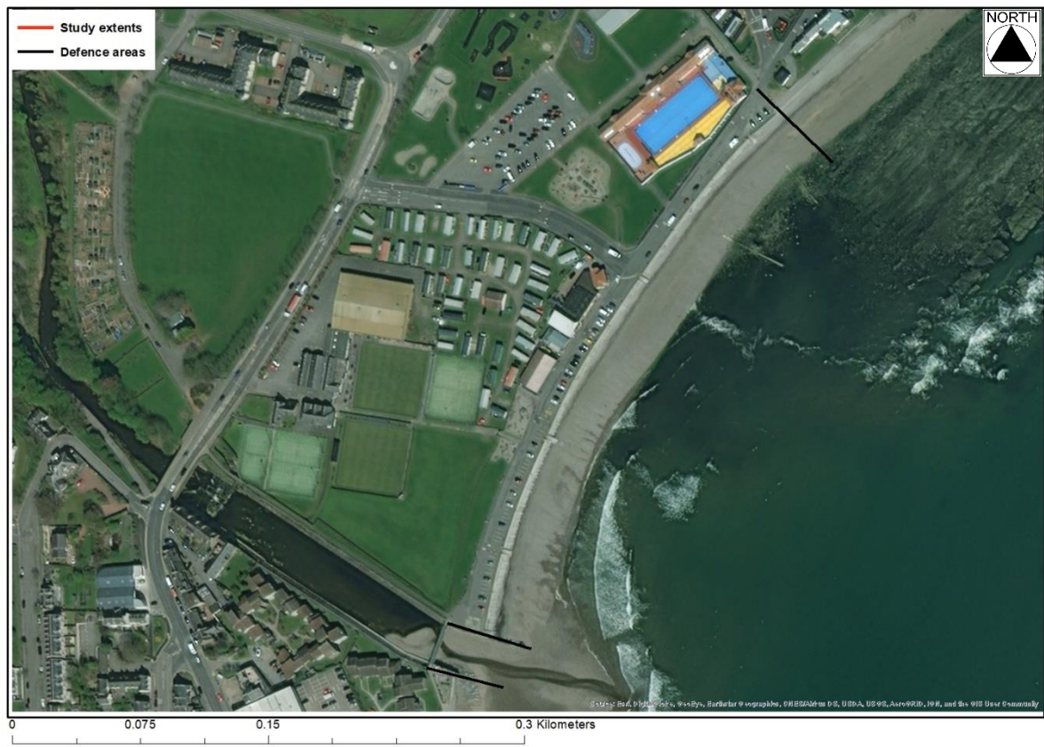
Figure 2-8: Aerial image of the stepped revetment section
