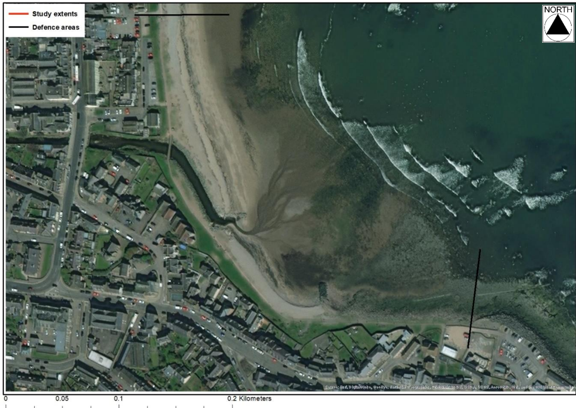
Figure 2-5: Aerial image of the boardwalk section
