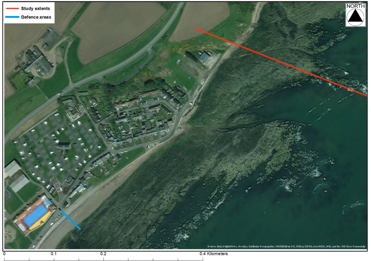
Figure 2-9: Aerial image of the Cowie wall section
