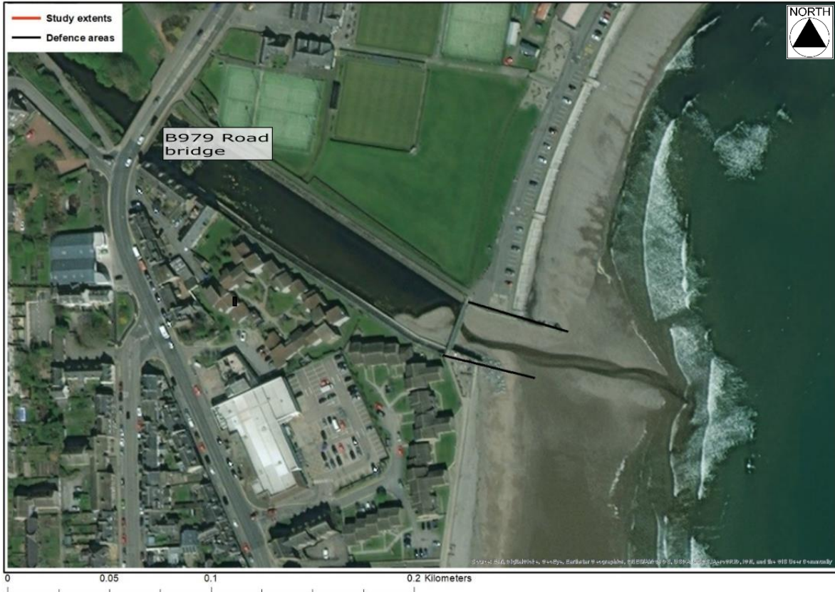
Figure 2-7: Aerial image of the River Cowie section
