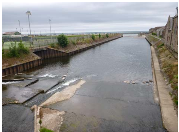
Plate 15 View from Cowie Bridge, looking east
