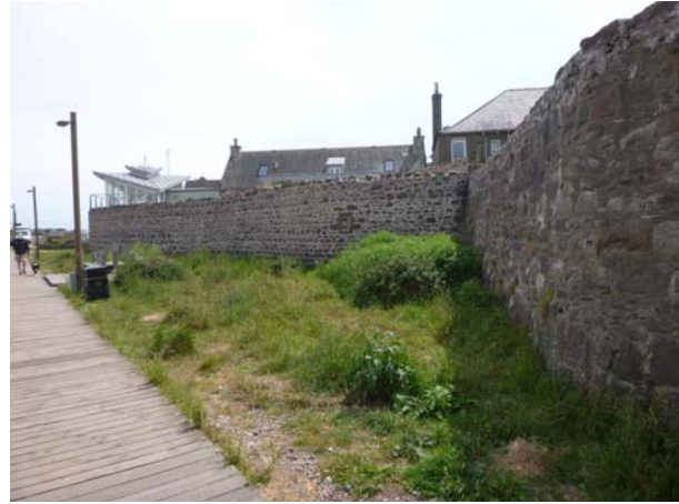
Plate 20 View of seawall to rear of Keith Place
