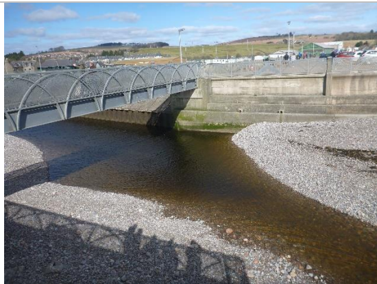
C: Looking downstream across the River Cowie. Narrowing of the channel outlet due to sedimentation.
