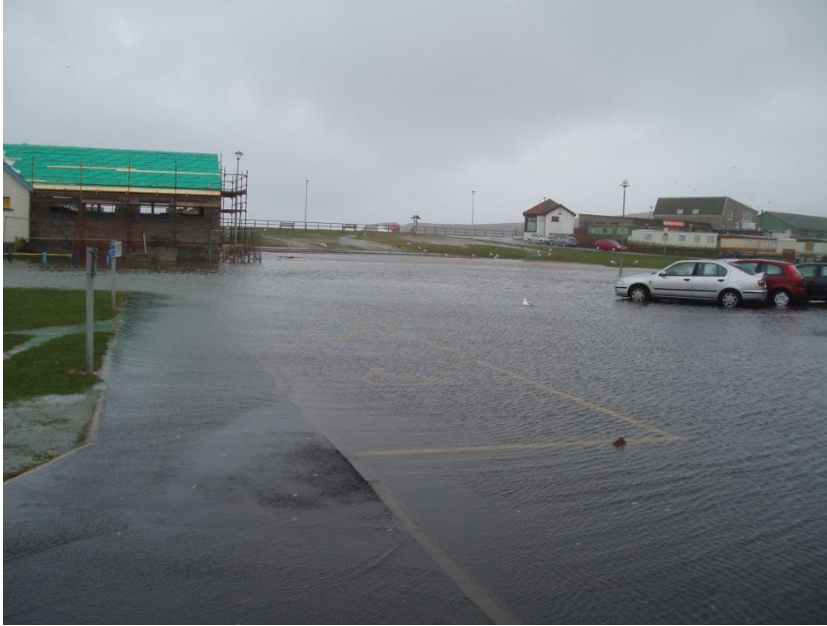
Flooding of car park behind swimming pool due to overland flow from overtopping of Cowie promenade. Photograph supplied by Aberdeenshire Council.
