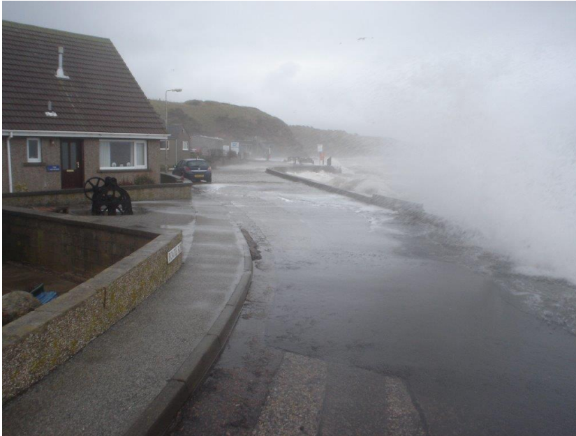
Overtopping of wall at Cowie village. Photograph supplied by Aberdeenshire Council.
