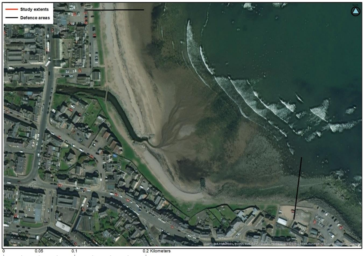
Figure 4-4: Aerial image of boardwalk section
