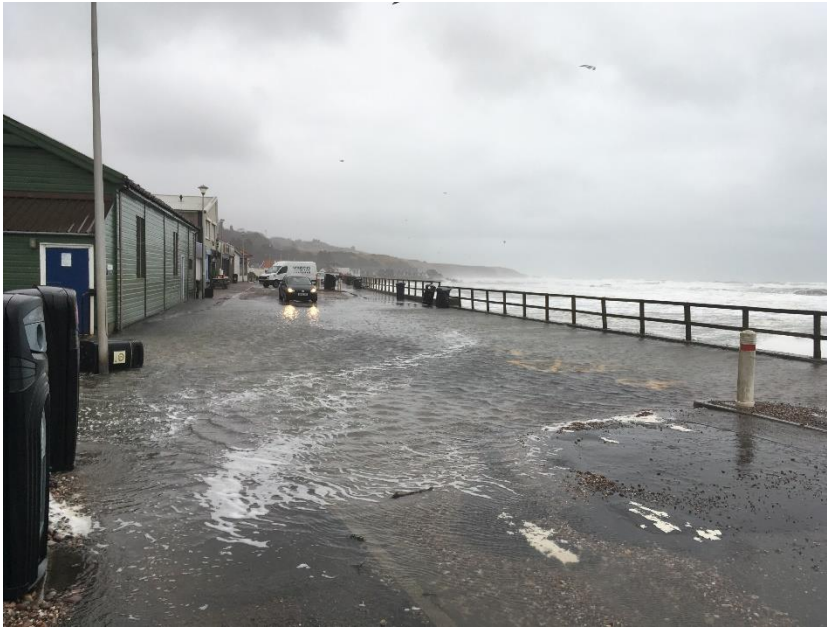
Overtopping at Cowie promenade. Photograph supplied by Aberdeenshire Council.
