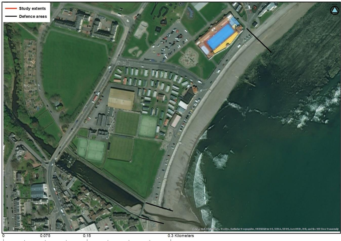
Figure 4-10: Aerial image of stepped revetment section
