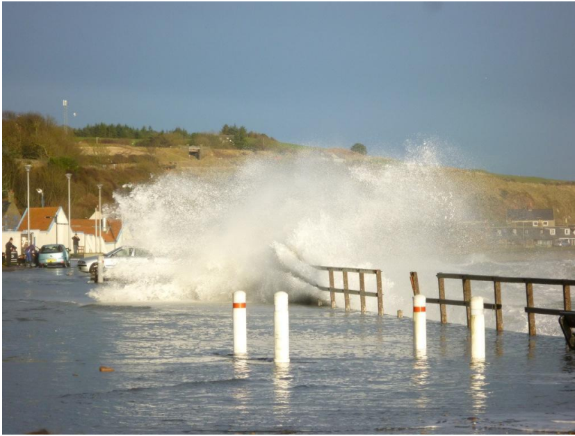
Overtopping of stepped revetment at Cowie promenade. Photograph supplied by Aberdeenshire Council.
