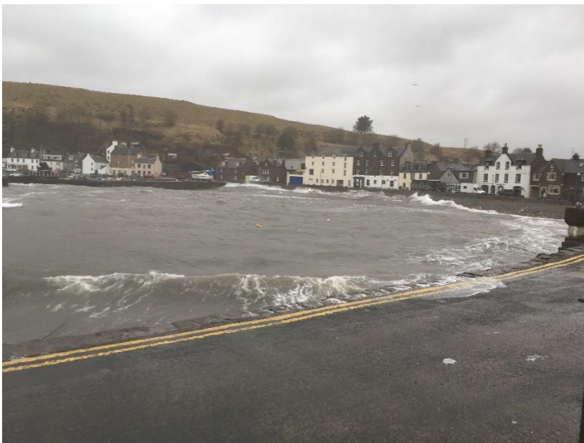
Wave action within the harbour. Photograph supplied by Aberdeenshire Council.
