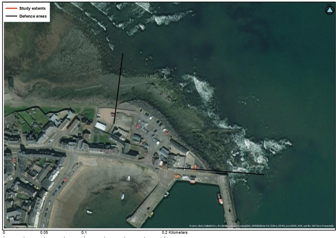
Figure 4-3: Aerial image of rock armour section
